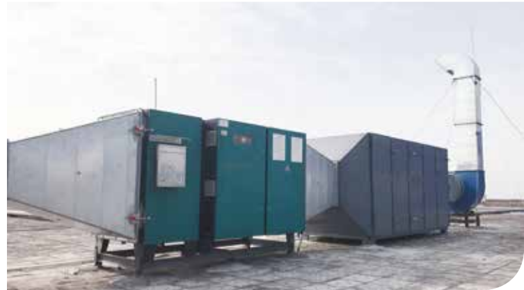
VOCs Emission Control Facility
