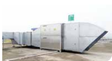
VOC Control Facilities
