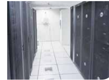
Computer Server Room
