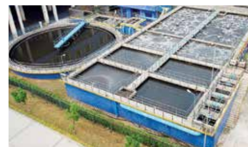
Wastewater Treatment Plant
