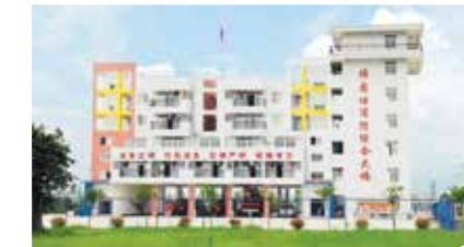
Leo Fire Fighting Building
