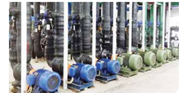
Slurry Ice Air-conditioning System Refrigeration pump & Cooling pump
