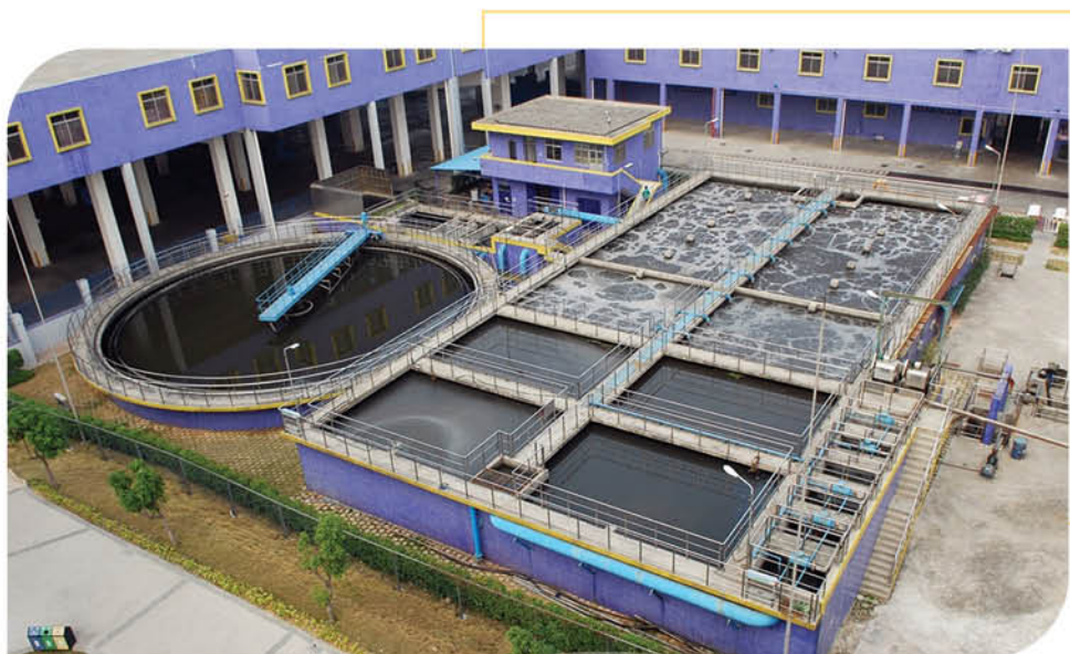
Waste water treatment plant
