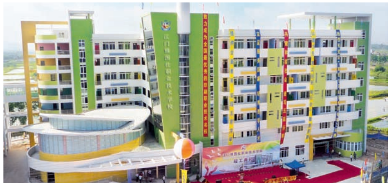
Energy-saving demonstrative project - Astros Vocational and School
